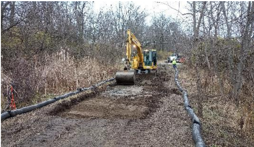
Building construction entrance from Sarah Bolton Park
