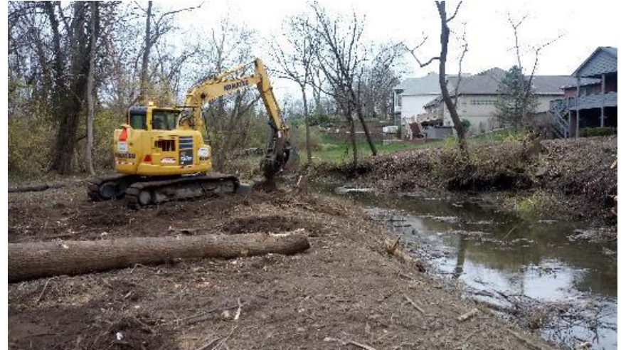
Clearing debris, west of the creek at STA: 29+00
