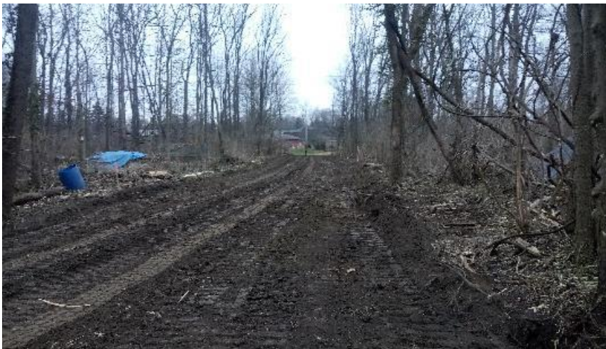
STA: 159+00, looking south at cleared path for the trail.
