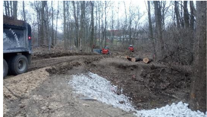
Clearing west toward the creek, around the bend at STA:159+00 to 161+00.
