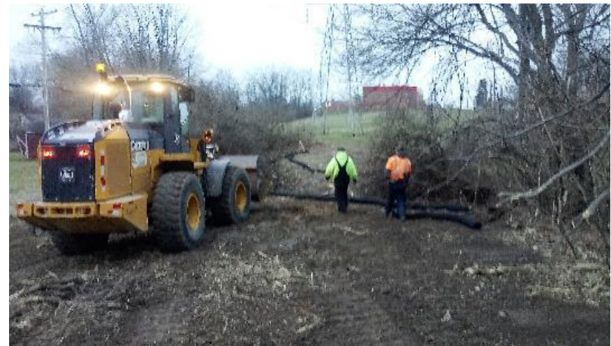
Installing filter sock at Beech Creek, location for Bridge #4.
