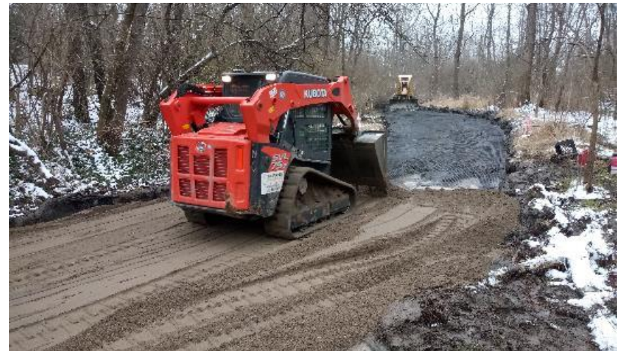
Skidsteer placing sand B borrow over geo-grid for subgrade treatment.
