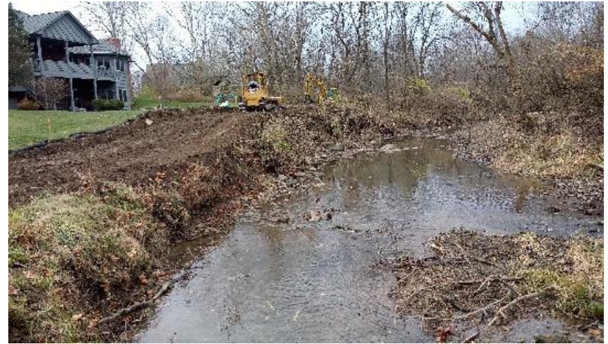
Dozing topsoil off to prepare for temporary construction access.
