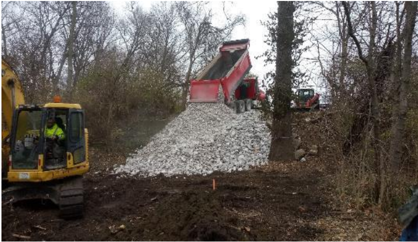
Placing riprap for temporary construction access from Sarah Bolton park.
