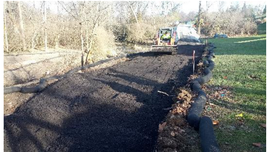
Skidsteer placing asphalt millings for the temporary access path.
