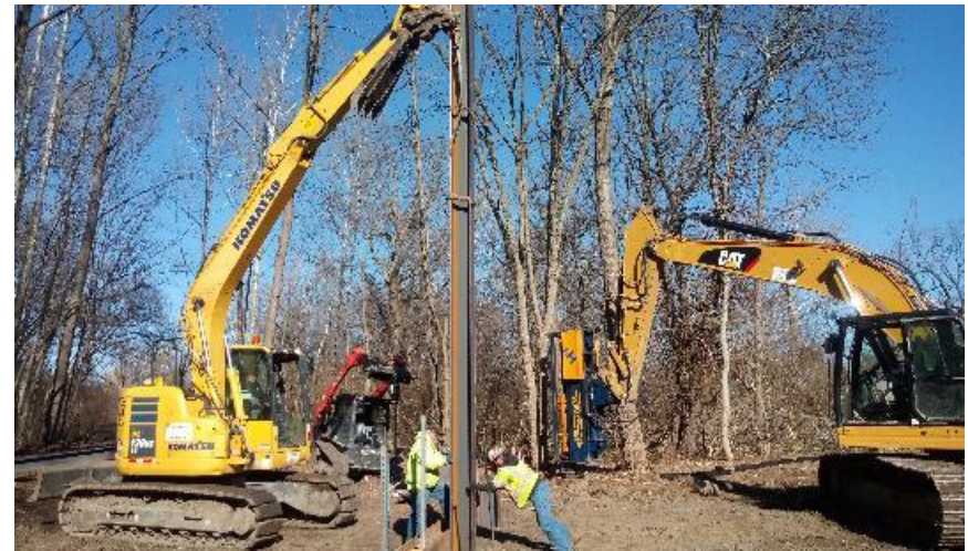
Lining up the steel pile for Bridge #4, bent # 2.
