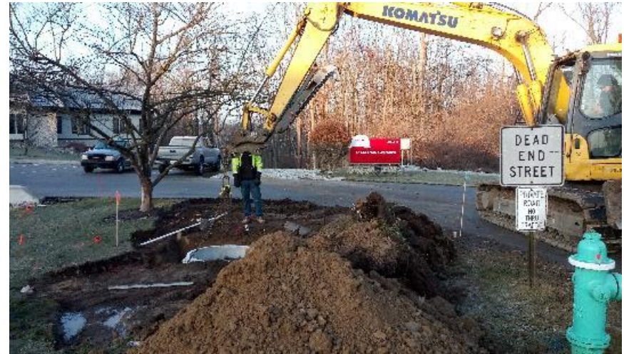
Setting the manhole at STA: 164+75 at the end of Hornet Avenue.
