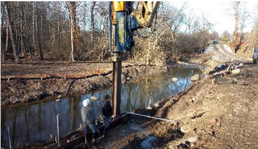
Preparing to drive the steel pile in Bridge #2, bent #1.
