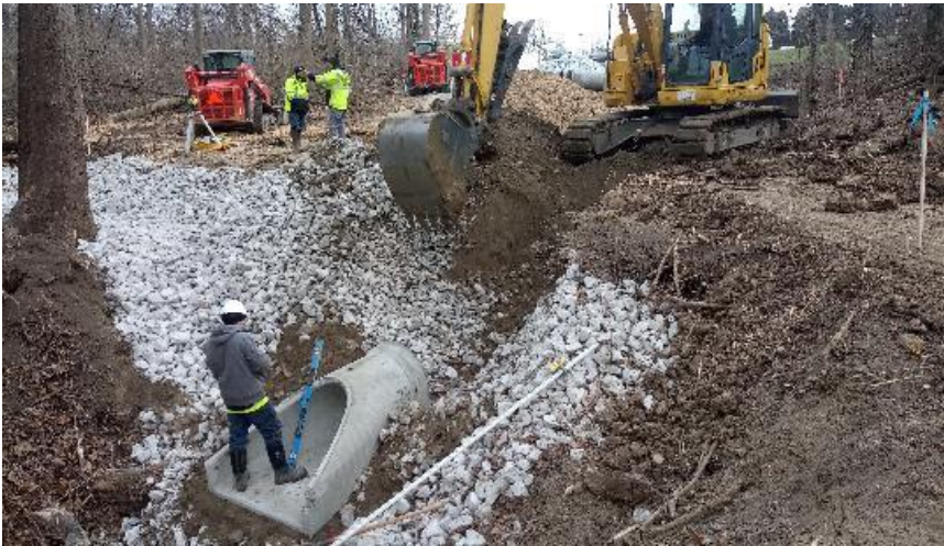
Setting end section at STA: 162+00 north of the Skillman building.
