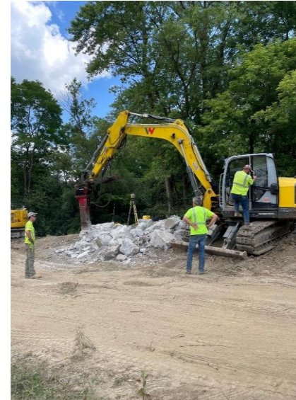
breaking large pieces of excavated concrete
