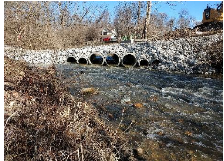
Constructing the stream crossing at Bridge #3.
