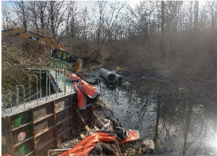
Constructing the stream crossing at Bridge #3.
