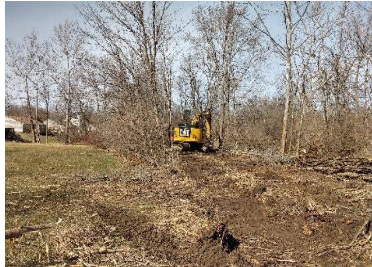
West side of Lick creek, clearing north toward Bridge #1.
