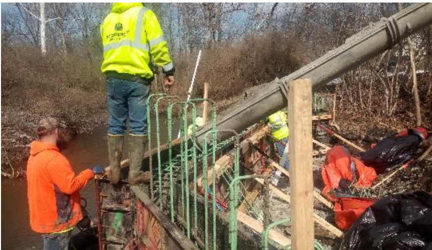
Pouring concrete for end bent #2 at Bridge #3.
