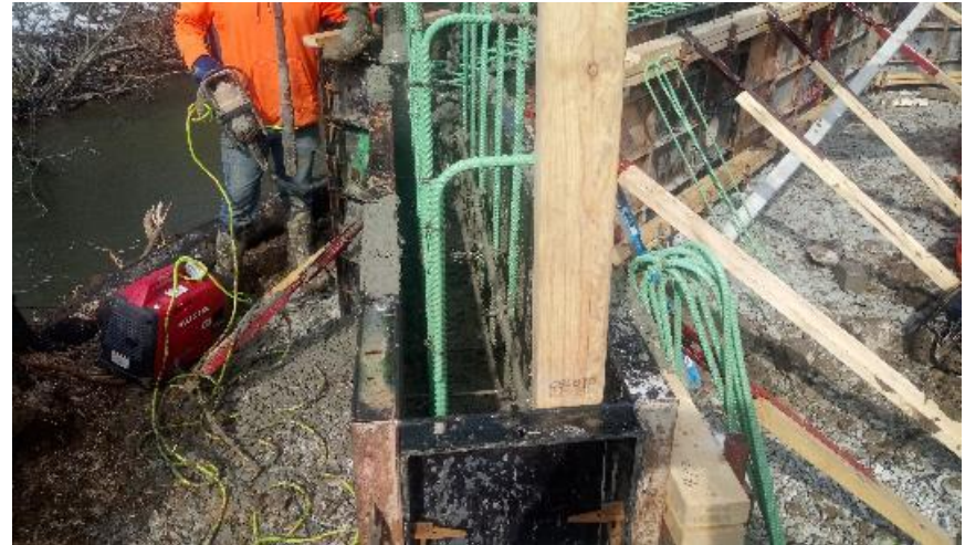
Pouring concrete for end bent #2 at Bridge #3.
