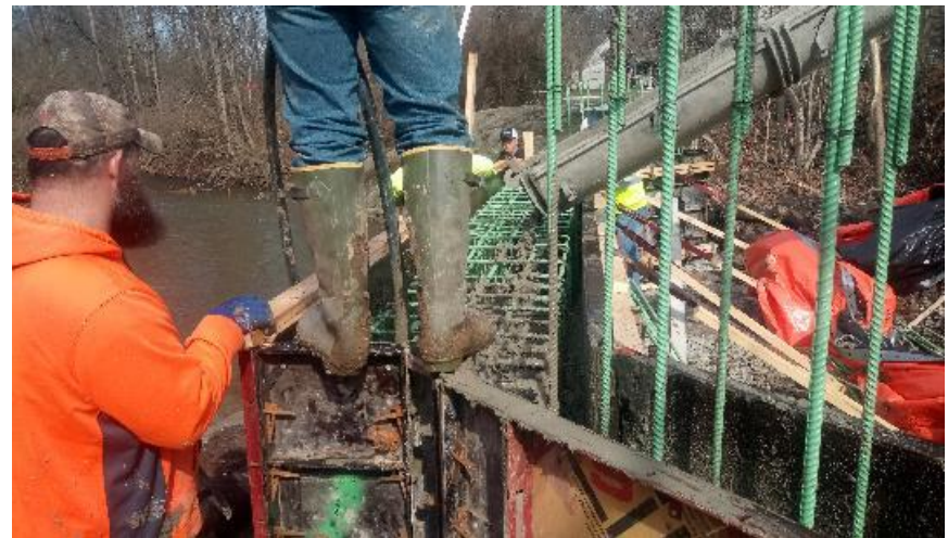
Pouring concrete for end bent #2 at Bridge #3.
