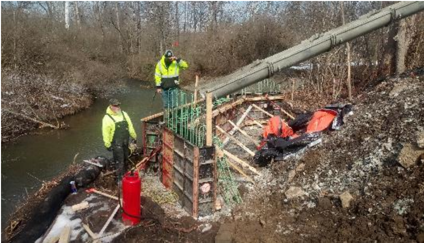
Pouring concrete for end bent #2 at Bridge #3.
