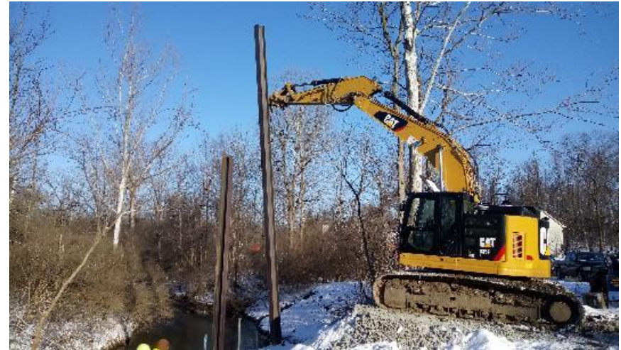
Excavator on built up ramp, placing the pile for Bridge #3, bent #2.
