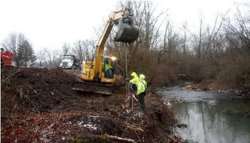
Preparing the area of bent #2, Bridge #3 for pile driving.
