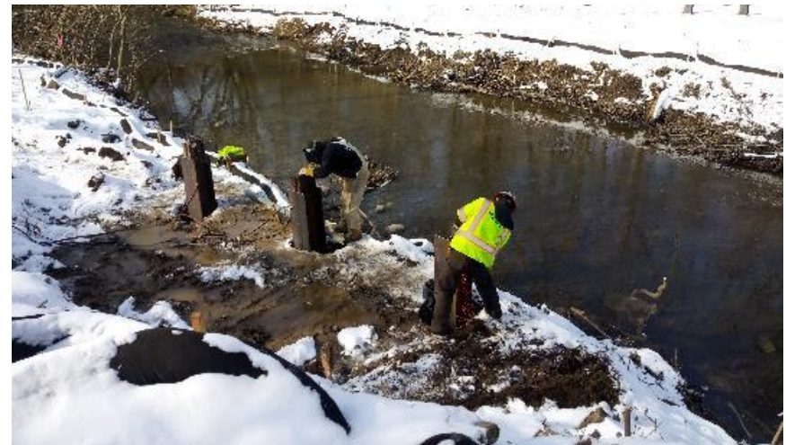
Morphey preparing the piles at Bridge #2, bent #2 for splicing.
