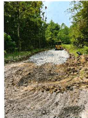
Stone going over sand for undercut West of bridge 3
