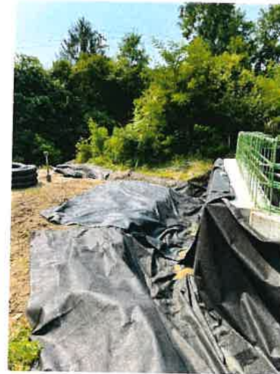
Fabric for underdrain bridge 4
