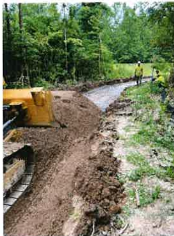
Placing Sand over Geo Grid for undercut West of bridge 3
