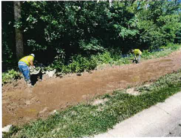
Pumping water and cutting trenches to facilitate drainage on Charnwood
