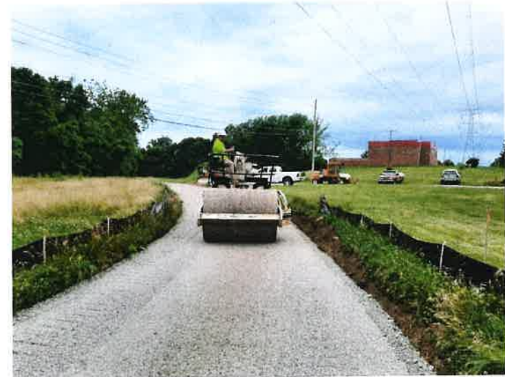
Rolling aggregate behind school towards bridge 4
