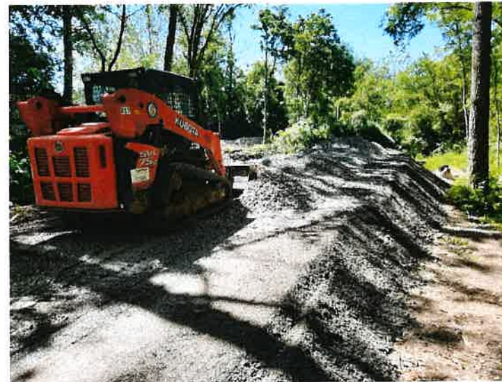
Placing aggregate over embankment Bridge 2
