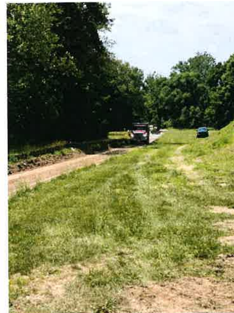
Placing aggregate headed to Bridge 4 from the Challis Park
