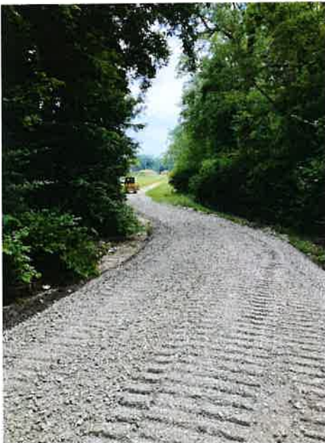
Going down the hill from Challis Park to Bridge 4
