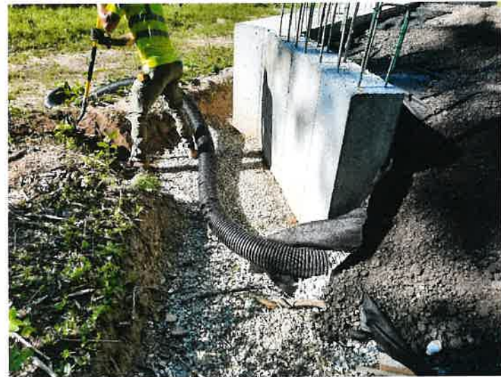
Underdrain at Bridge 2
