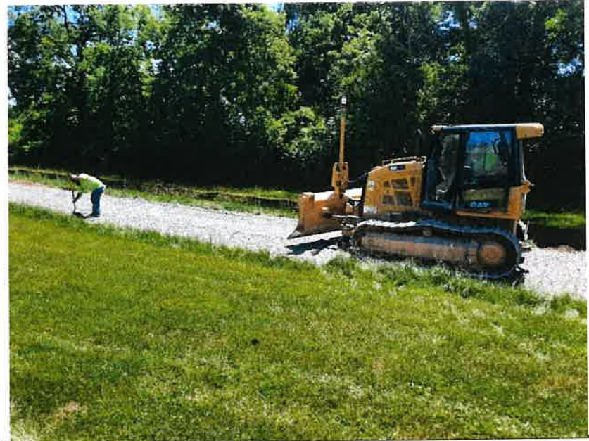
Placing aggregate in Challis Park
