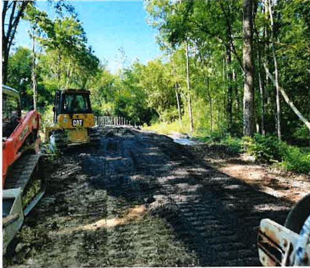
Placing and rolling embankment to Bridge 2
