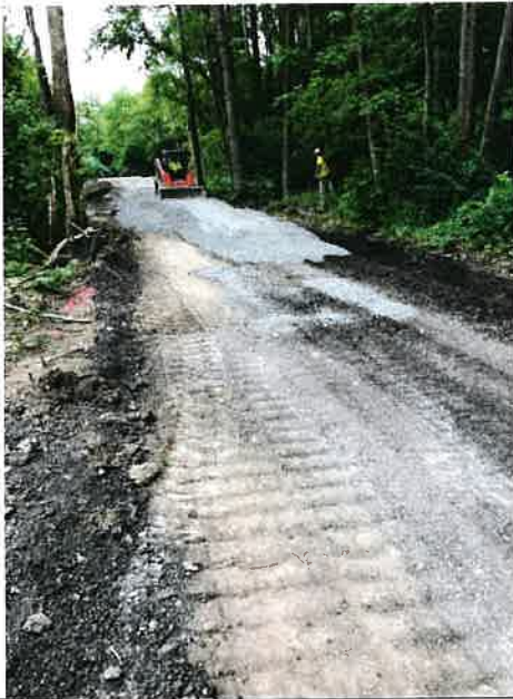
Aggregate placement Bridge 2
