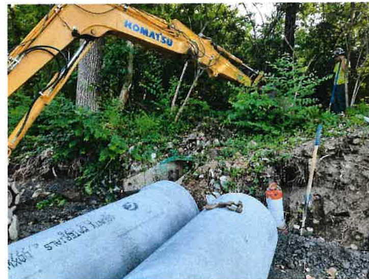
Existing drainage structure North of bridge 1
