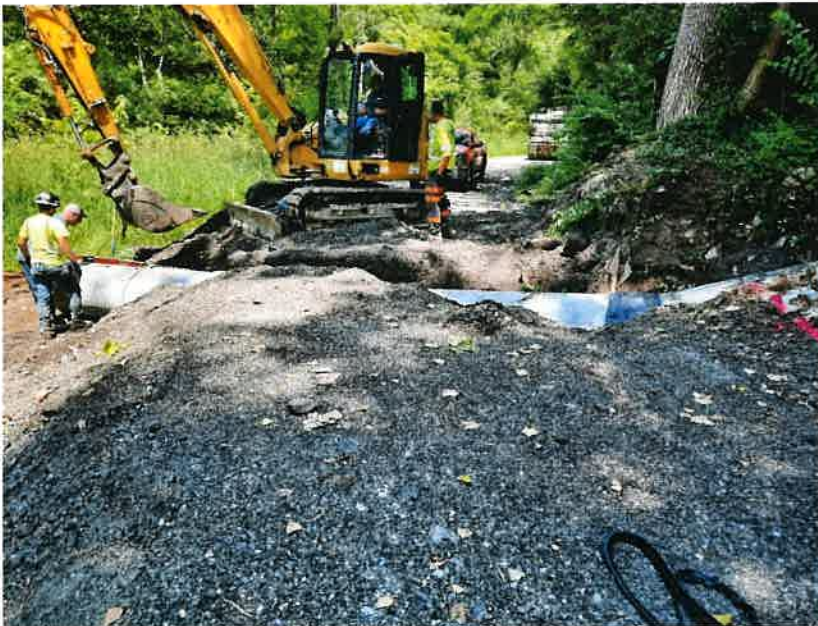
Placing last section of pipe
