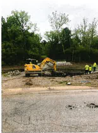
Clearing debris along the stream crossing
