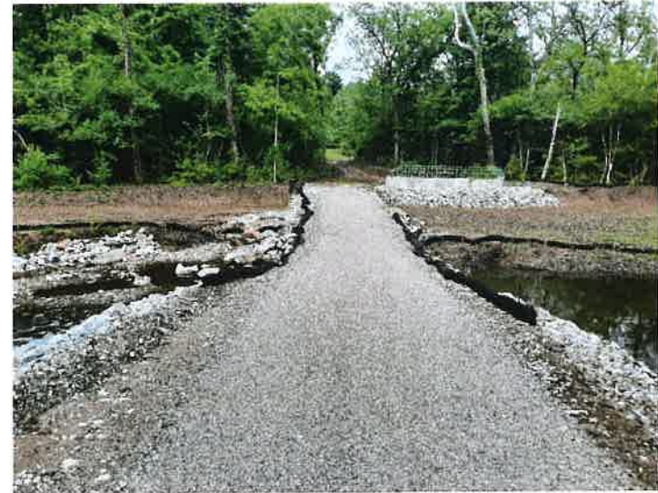
Repaired stream crossing
