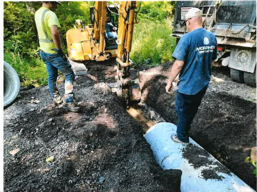
Crossing the path with pipe
