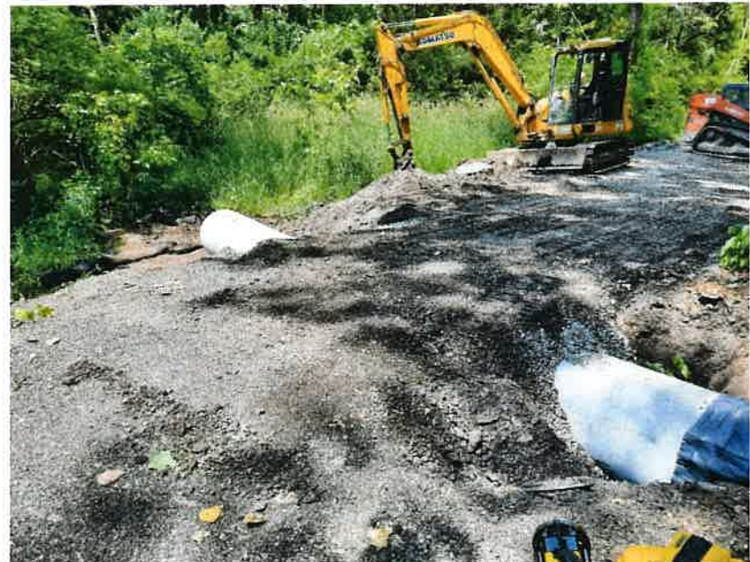
Backfilling pipe crossing
