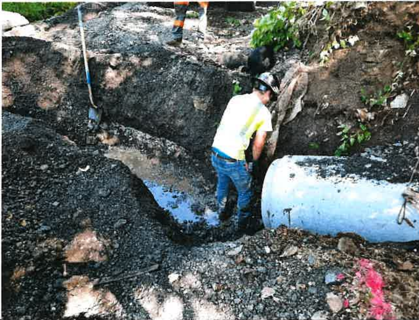
Tying into existing structure
