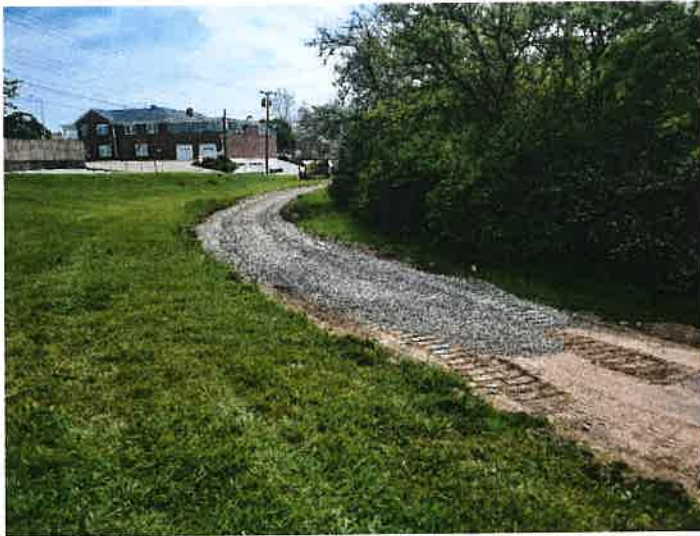
Placing compacted aggregate in Bolton Park
