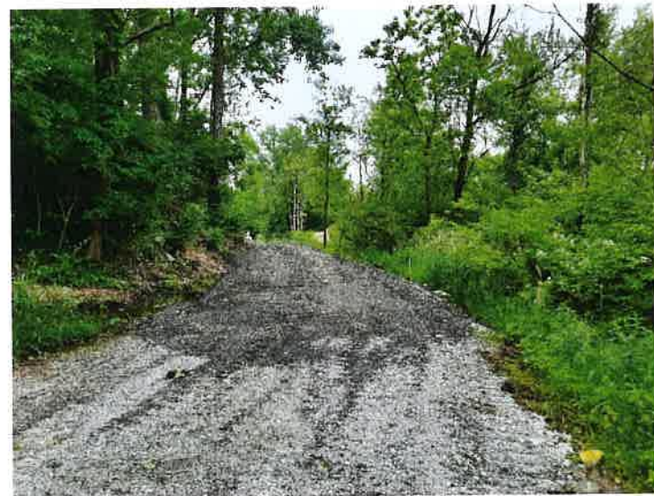
Fill area leading to bridge 1
