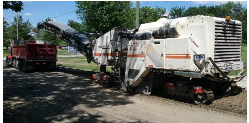
Milling for full depth road removal on Butler Avenue.
