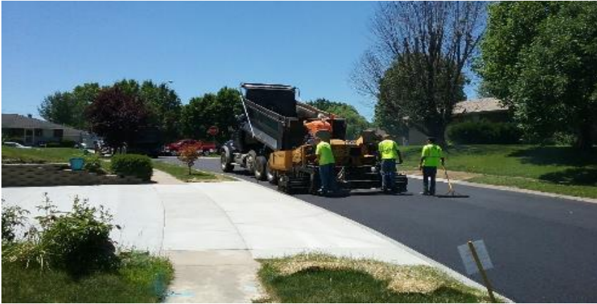
Placing surface asphalt on Birch Street.
