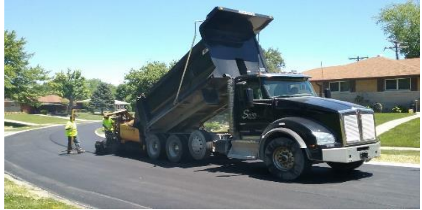
Placing surface asphalt on Birch Street.
