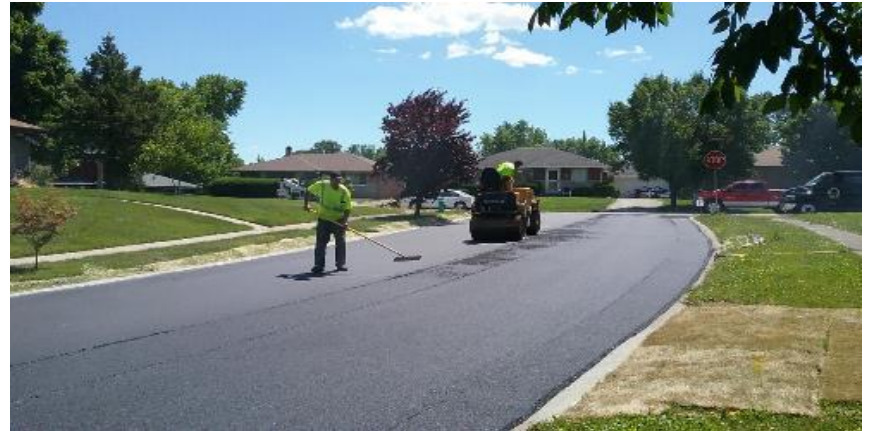
Roll compacting surface asphalt on Birch Street.
