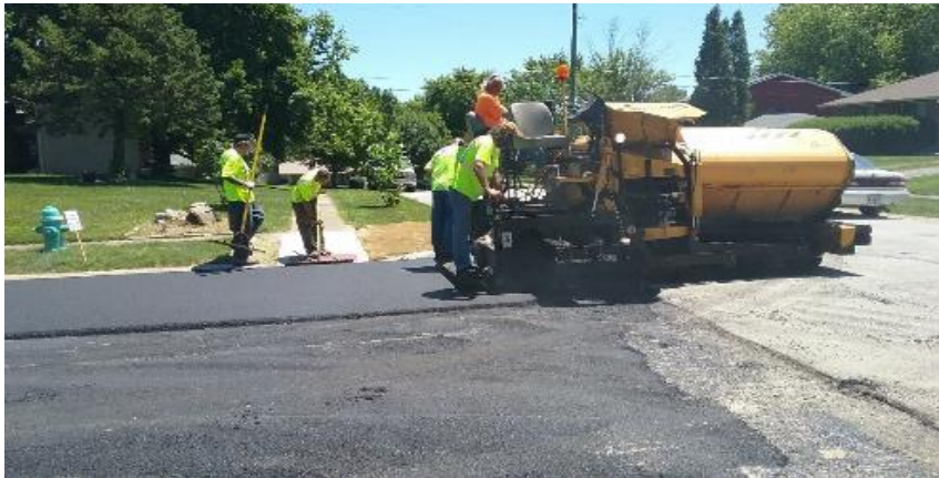
Placing surface asphalt on Birch Street.
