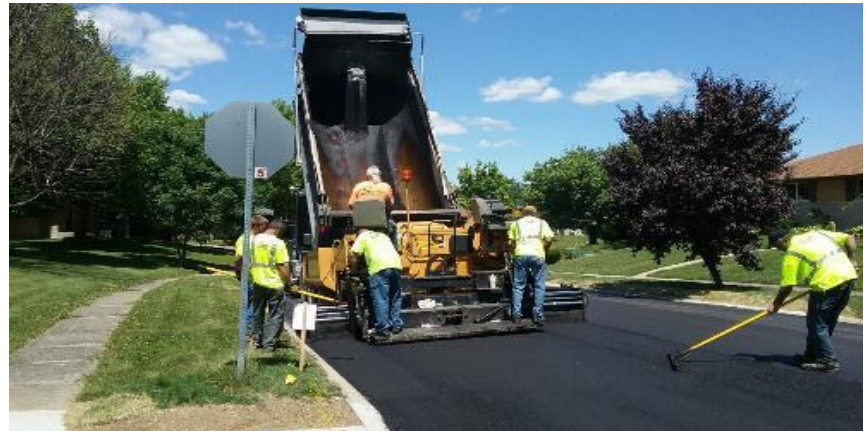
Placing surface asphalt on Birch Street.
