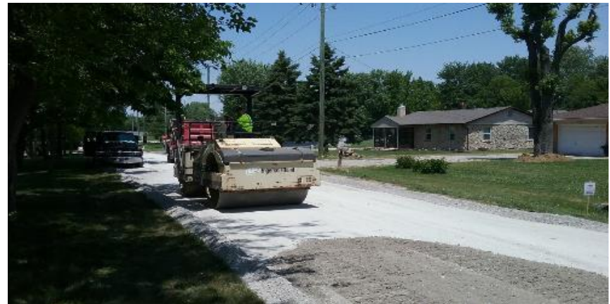
Roll compacting stone for subgrade treatment on Butler Avenue.
