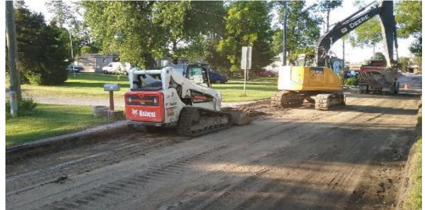
Grading subbase on Butler Avenue.
