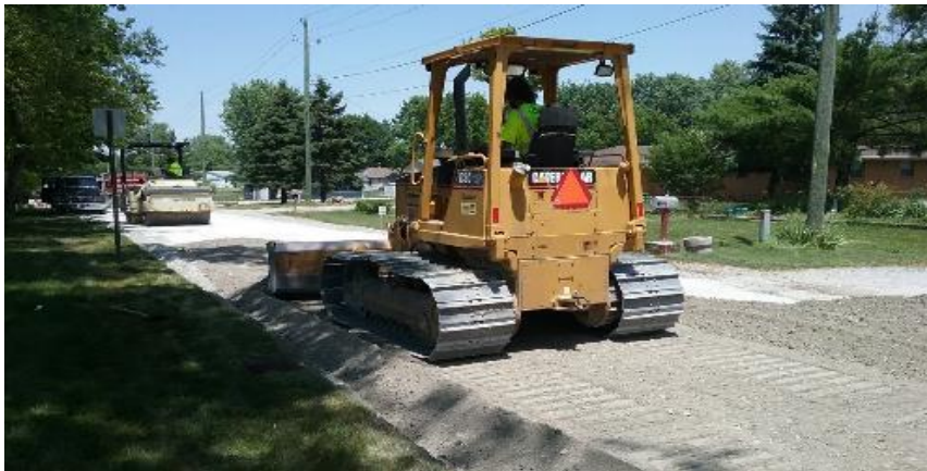
Grading stone for subgrade treatment on Butler Avenue.
