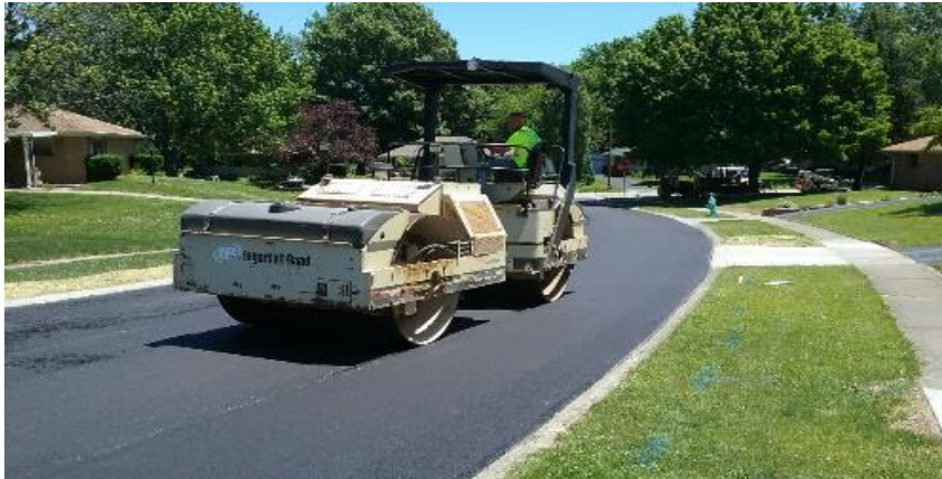
Roll compacting surface asphalt on Birch Street.
