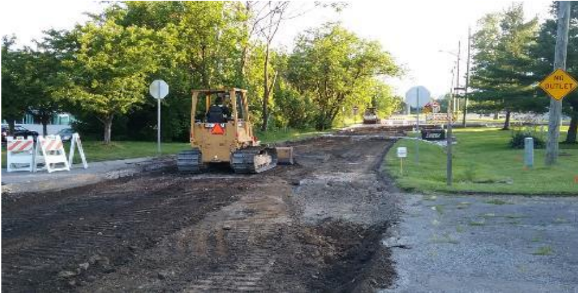
Grading subbase on Butler Avenue.
