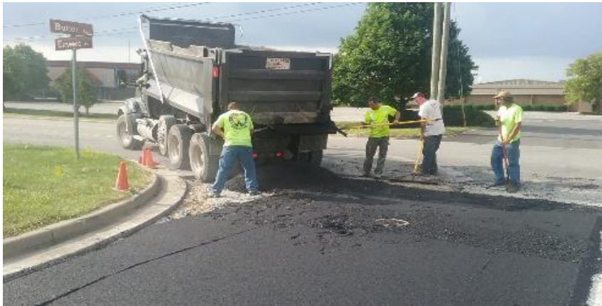
Placing intermediate asphalt on Butler Avenue.
