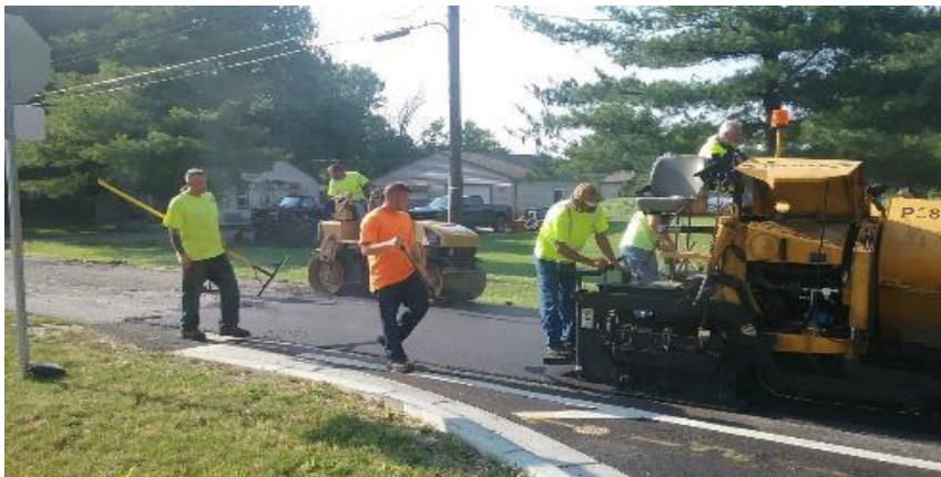
Placing surface asphalt on Butler Avenue.
