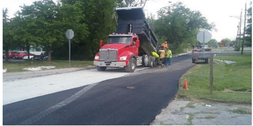
Placing intermediate asphalt on Butler Avenue.
