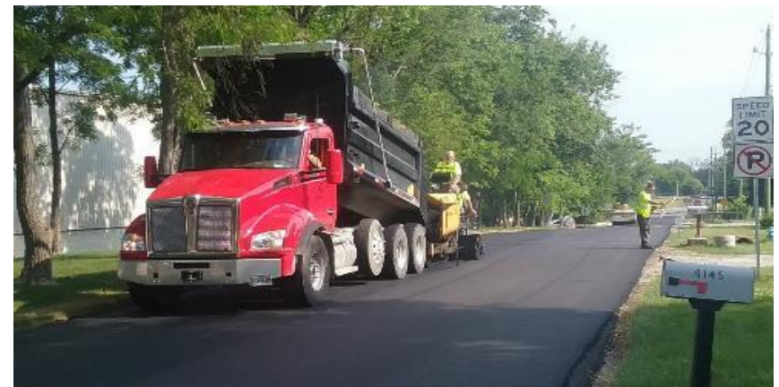
Placing surface asphalt on Butler Avenue.
