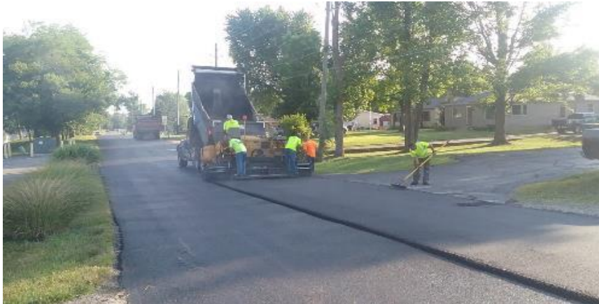
Placing surface asphalt on Butler Avenue.
