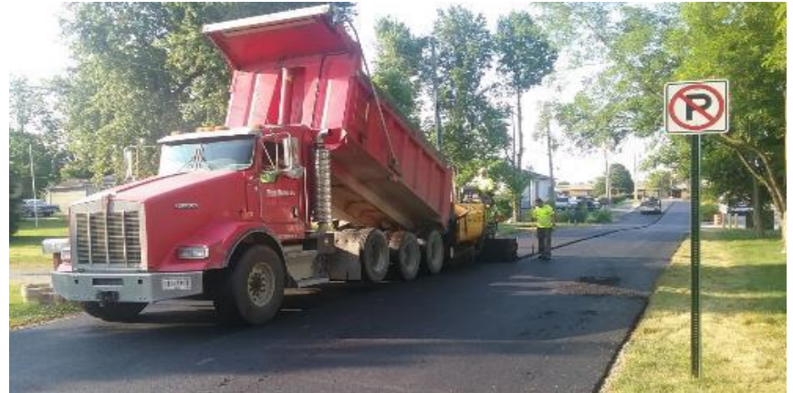
Placing surface asphalt on Butler Avenue.
