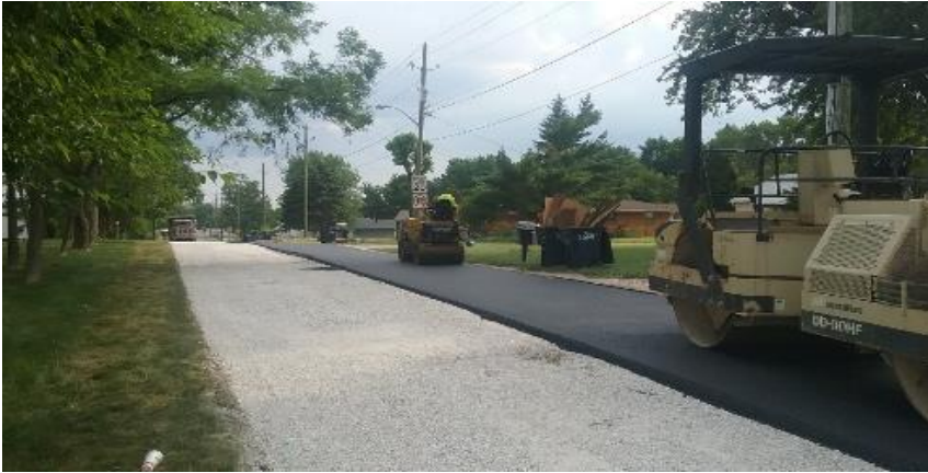
Roll compacting intermediate asphalt on Butler Avenue.
