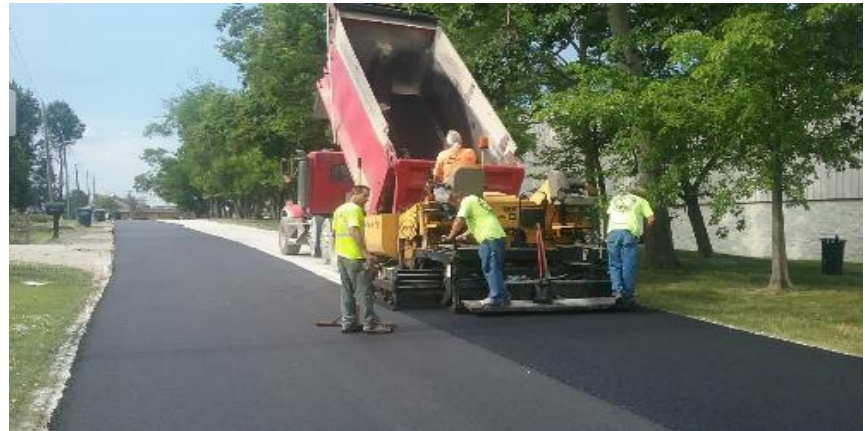
Placing intermediate asphalt on Butler Avenue.
