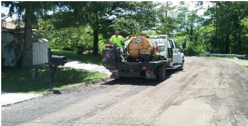
Placing tack down for asphalt paving on Lifegate Way.
