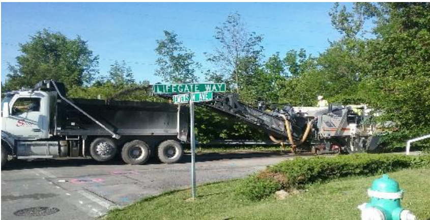
Milling on Lifegate Way at Emerson Avenue.
