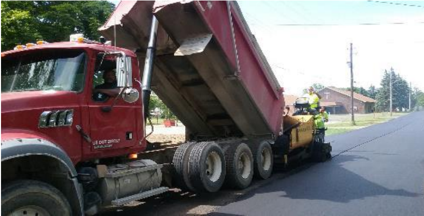
Paving surface asphalt on Lifegate Way.
