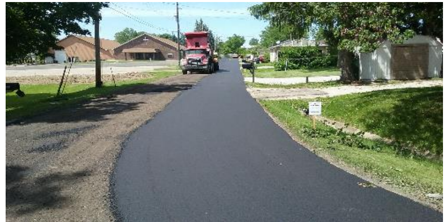
Paving surface asphalt on Lifegate Way.
