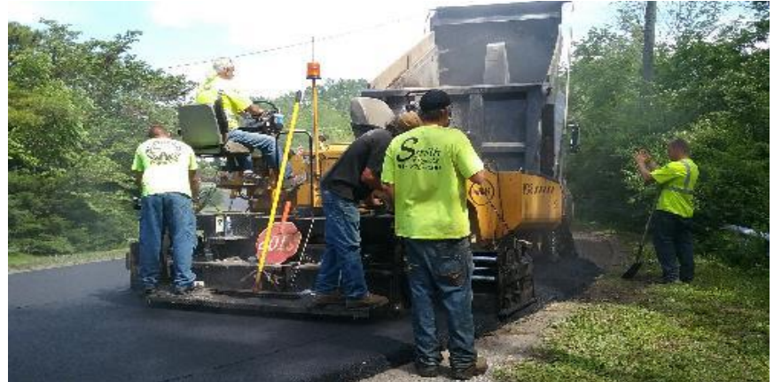
Paving surface asphalt on Lifegate Way.
