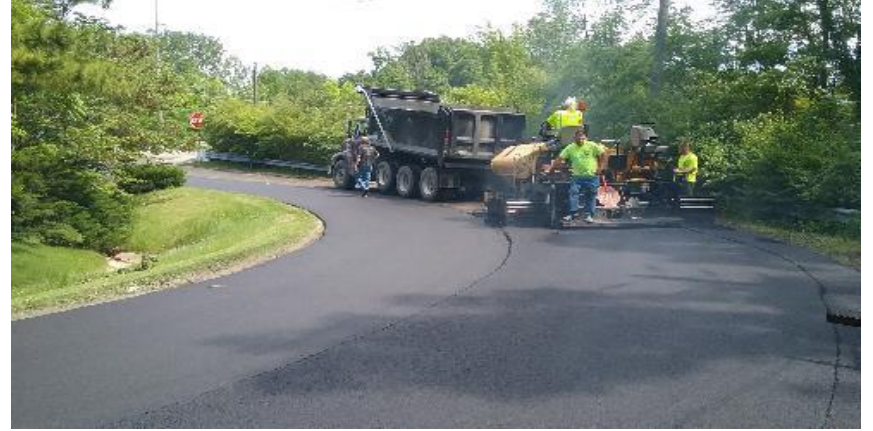
Paving surface asphalt on Lifegate Way.
