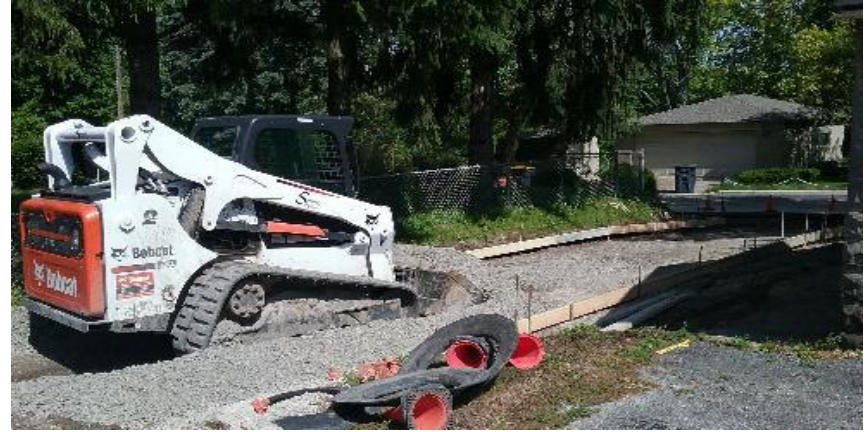
Placing stone subgrade alley approach, Southeast Pkwy, between 11th & 12th.
