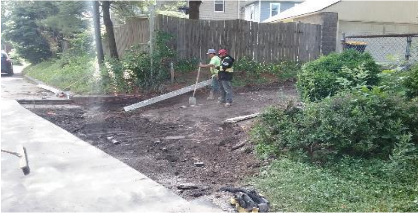
Removing alley approach on Southeast Pkwy, between 11th and 12th.
