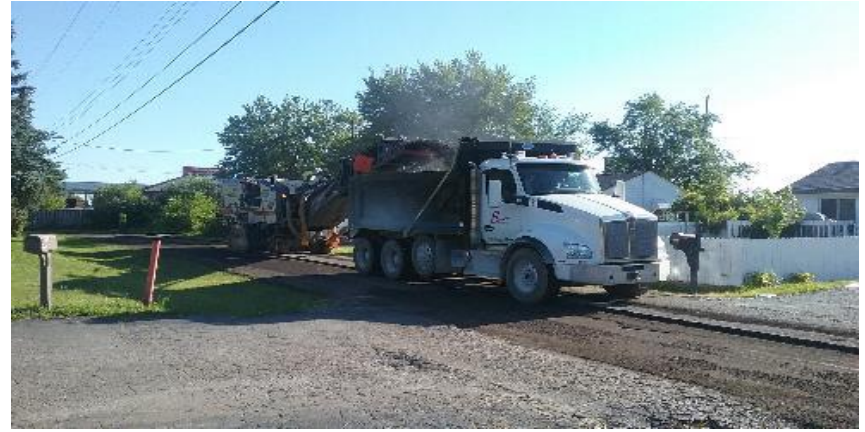
Milling on Lifegate Way.
