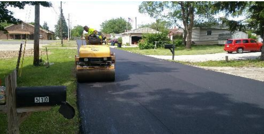
Roll compacting surface asphalt on Lifegate Way.
