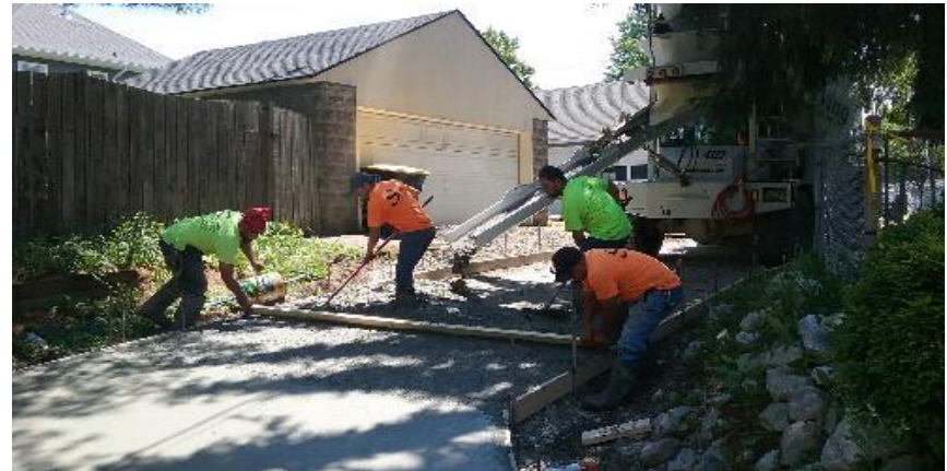
Pouring concrete alley approach on Southeast Pkwy, between 11th and 12th.
