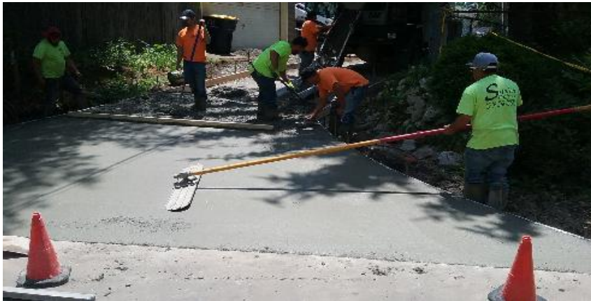
Finishing concrete alley approach on Southeast Pkwy, between 11th and 12th.
