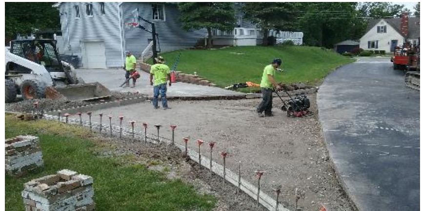
Forming, compacting alley approach, Southeast Pkwy between 12th and 13th.
