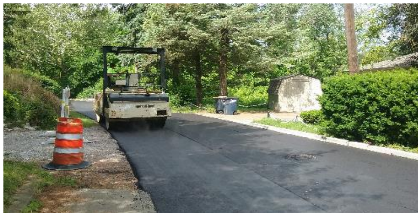
Roll compacting surface asphalt on Southeast Parkway.
