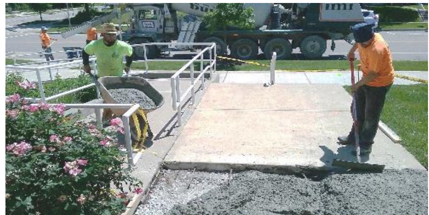
Placing concrete for new sidewalk ramp to City Hall.
