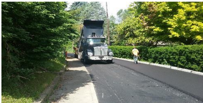
Placing surface asphalt on Southeast Parkway, just east of 12th Avenue.
