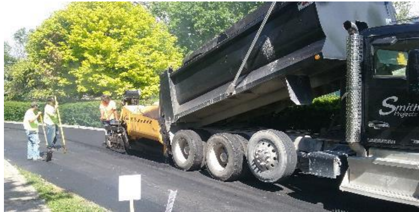
Placing surface asphalt on Southeast Parkway, just west of 11th Avenue.
