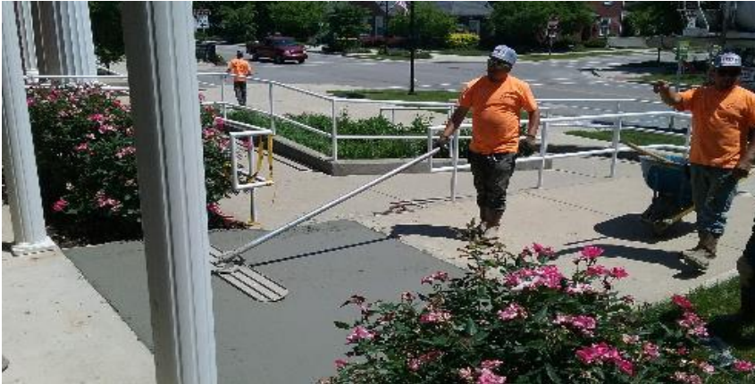
Finishing concrete for new sidewalk ramp to City Hall.
