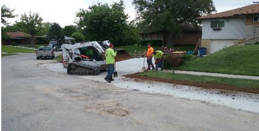
Backfilling dirt around curb and drive approached on Birch Street.
