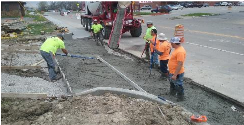
Pouring the driveway approach for first business lot, northside Churchman Ave.
