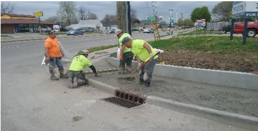
Striking off the concrete for sidewalk, corner of Emerson and Churchman.
