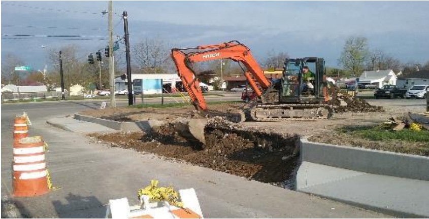
Excavating driveway approach for first business lot, northside Churchman Ave.
