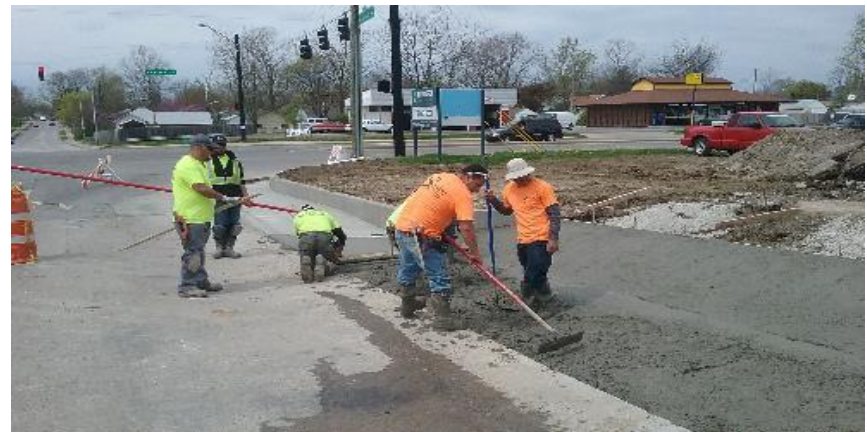
Finishing driveway approach for first business lot, northside Churchman Ave.
