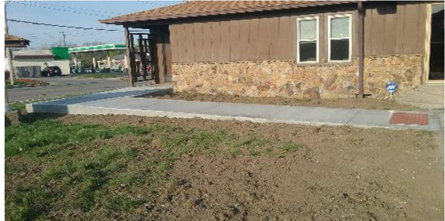
ADA ramp completed by Smith Projects on Henthorn property.
