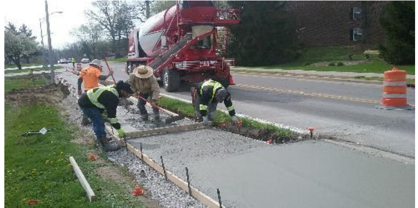
Striking off concrete sidewalk east of Senior facility northside Churchman Ave.
