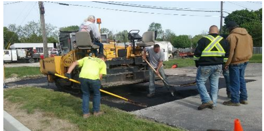
Placing surface asphalt at the Henthorn lot.
