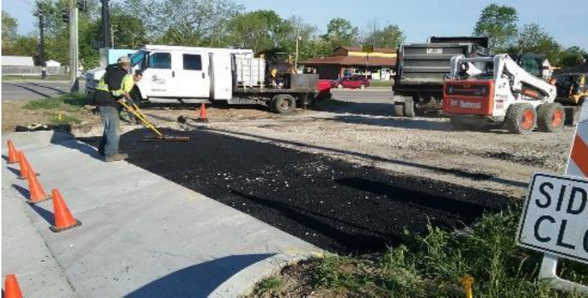
Asphalt placed in the approach on Churchman Avenue.
