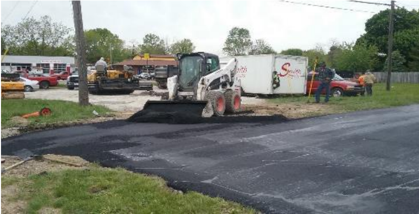
Forming asphalt edge for the Henthorn parking lot.
