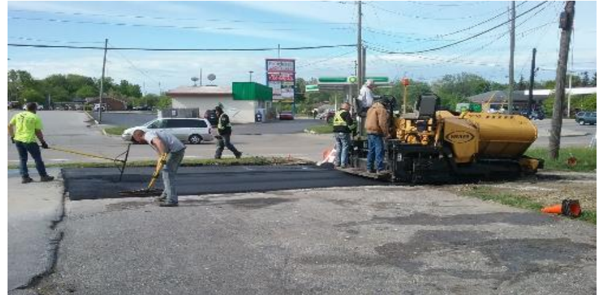
Placing surface asphalt at the Henthorn lot.
