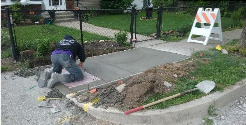
Finishing ADA ramp on northwest corner of 7th Avenue and alley.
