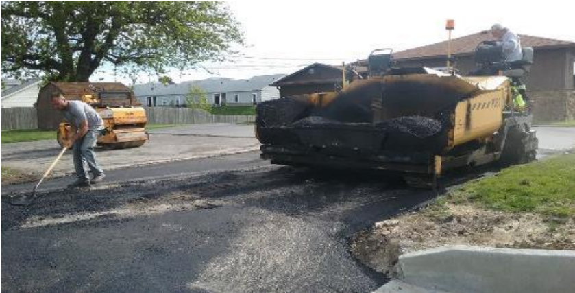
Placing surface asphalt at the Henthorn lot.
