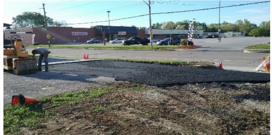
Asphalt for the Henthorn parking lot approach off of Churchman Ave.
