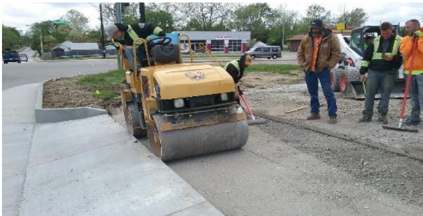
Compacting subgrade for the approach on Churchman Avenue.
