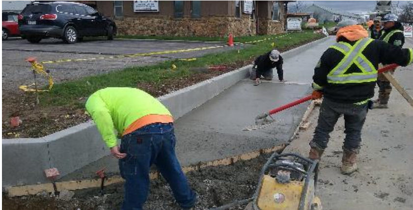
Finishing concrete sidewalk driveway transition north of Churchman Ave.
