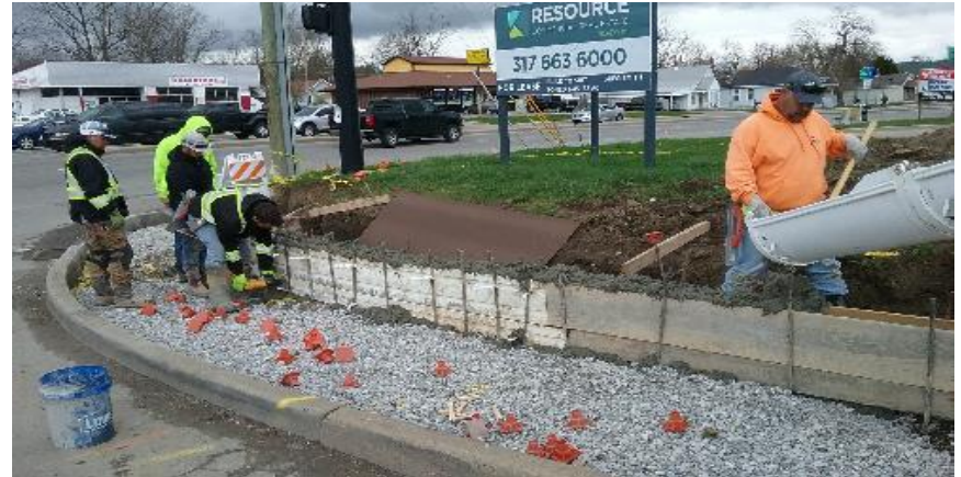
Pouring concrete for backside of sidewalk curb at Emerson and Churchman.
