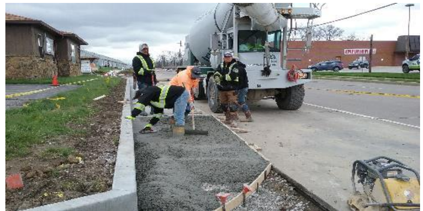
Pouring concrete sidewalk driveway transition north of Churchman Ave.
