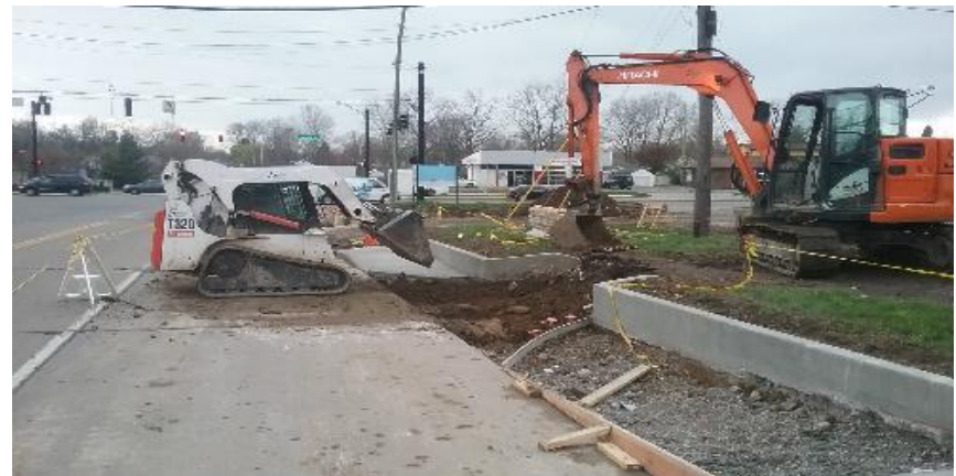
Excavating business drive approach for Henthorne property on Churchman.
