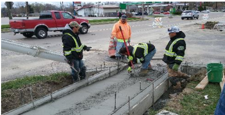
Pouring concrete ADA curb ramp east side of Schaff Street.
