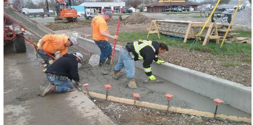
Pouring sidewalk between business approaches, north of Churchman.
