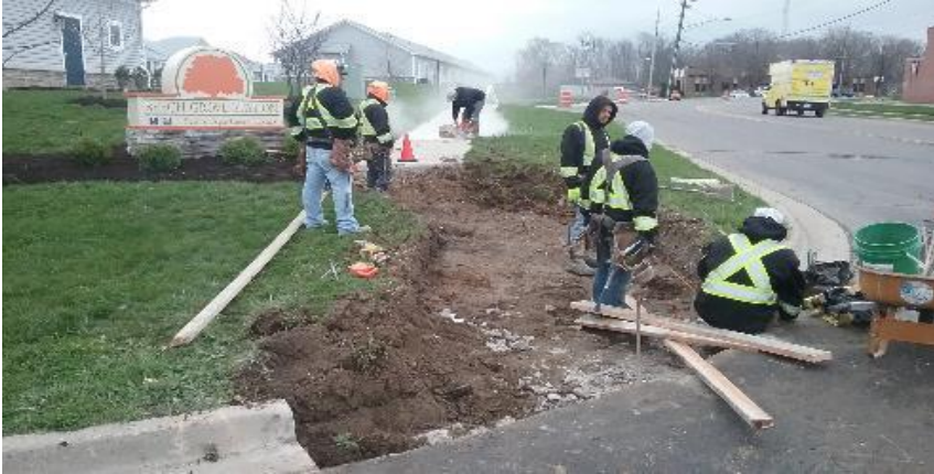
Forming ADA curb ramp, east of Schaff Street on Churchman Avenue.
