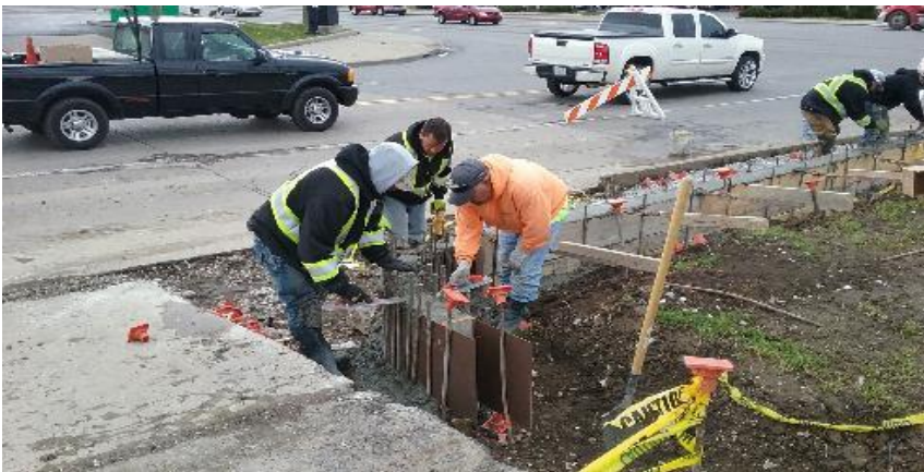
Pouring concrete, backside of sidewalk curb, first business drive on Churchman.
