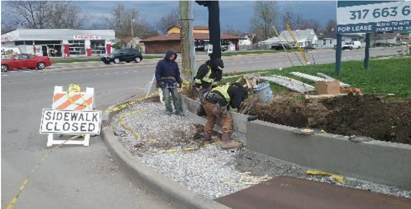
Forming backside sidewalk retaining curb at Emerson and Churchman.
