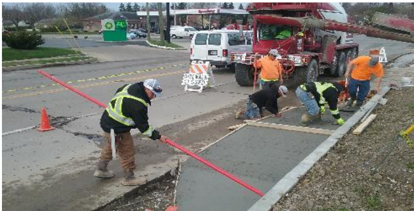
Finishing sidewalk between business approaches, north of Churchman.
