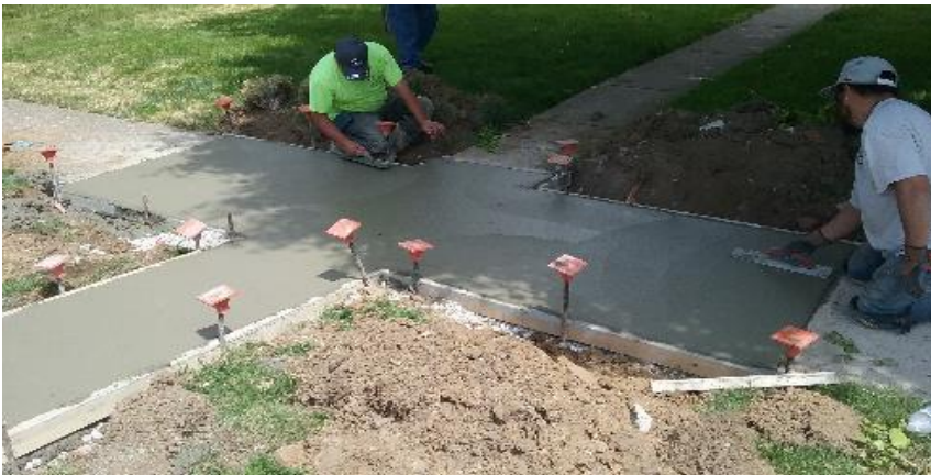
Finishing concrete sidewalk on the east side of N. 9th Avenue.
