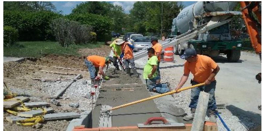
Pouring lowered concrete sidewalk approach at 174 N. 9th Avenue.
