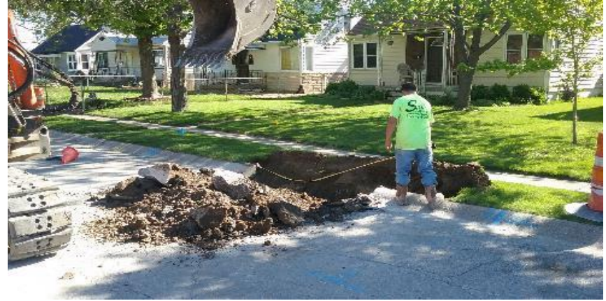
Removing existing curb to be replaced on N. 9th Avenue.
