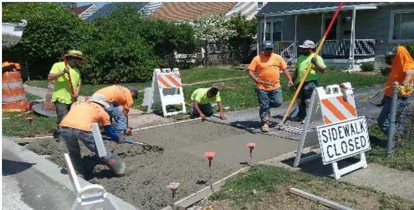
Pouring the concrete approach for 119 N. 9th Avenue.
