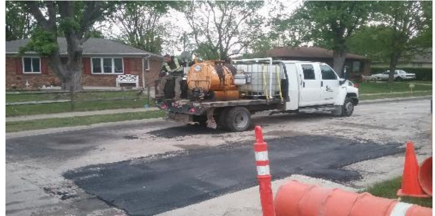
Placing tack on St. John's Court.
