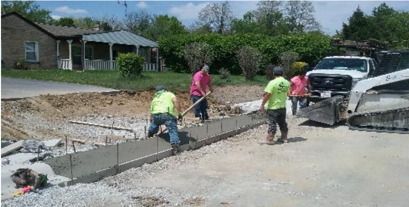
Finishing concrete curb and gutter at 174 N. 9th Avenue.
