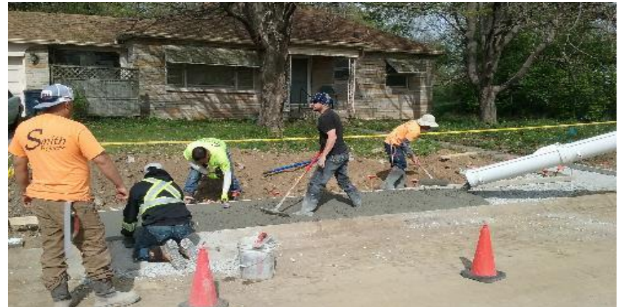
Pouring and finishing concrete sidewalk in front of 166 N. 9th Avenue.
