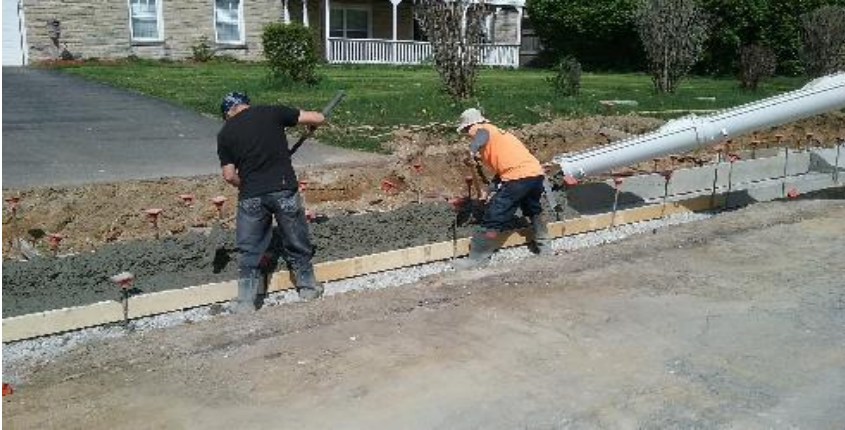
Pouring curb and gutter in front of 174 N. 9th Avenue.
