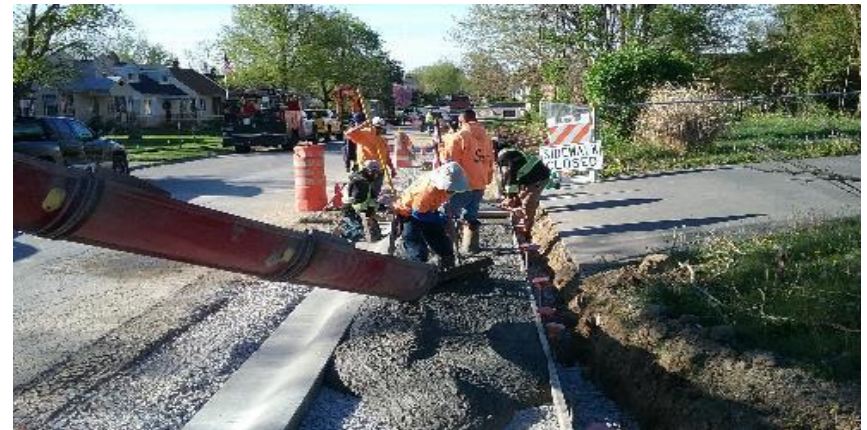
Pouring concrete sidewalk in front of home at 174 N. 9th Avenue.
