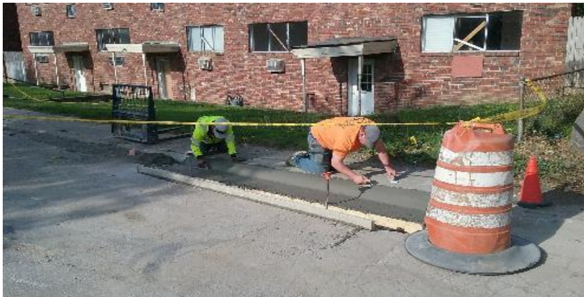
Edging concrete curb and gutter, west side of 9th Avenue.
