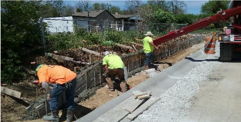
Pouring and finishing concrete modified curb at 174 N. 9th Avenue.
