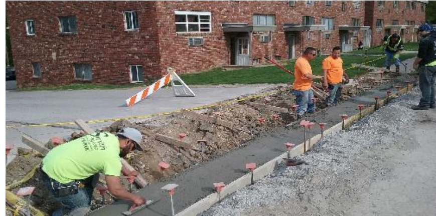
Finishing the concrete curb and gutter for Wilmar Apartments approach.
