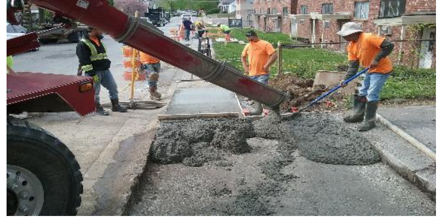
Pouring the concrete driveway approach for home at 166 N. 9th Avenue.
