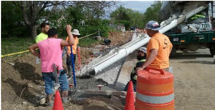
Pouring concrete sidewalk in front of home at 166 N. 9th Avenue.
