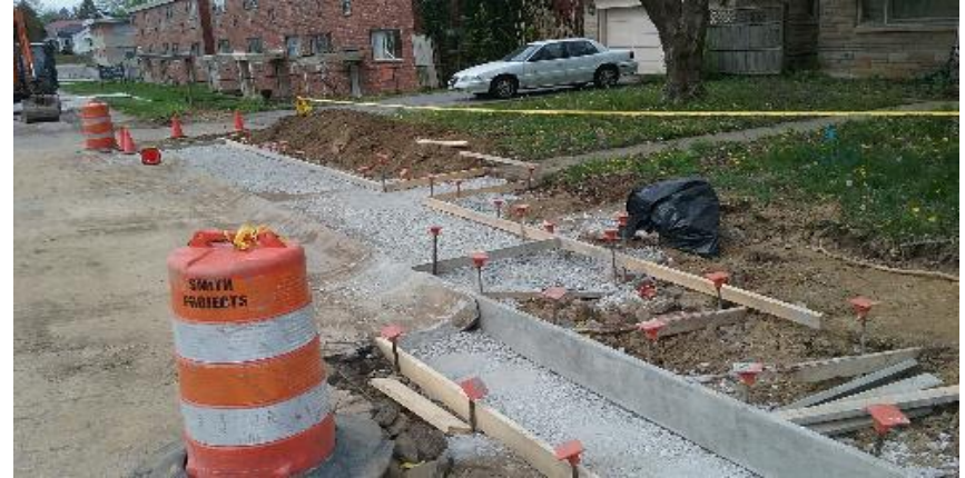
Curb and sidewalk formed up in front of 166 N. 9th Avenue.
