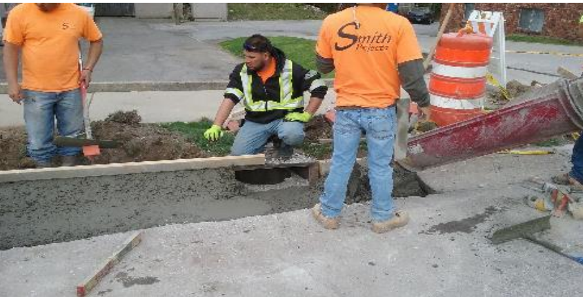
Forming curb flow line to the inlet west side of 9th Ave. just north of Albany St.
