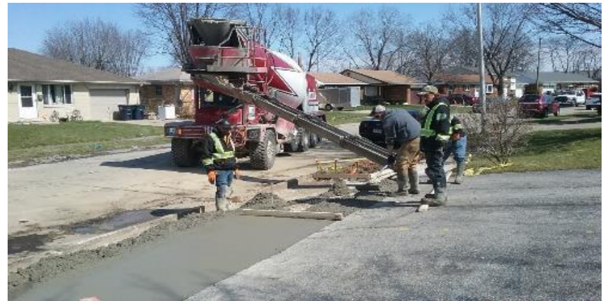
Pouring driveway approach at 515 St. John's Court.
