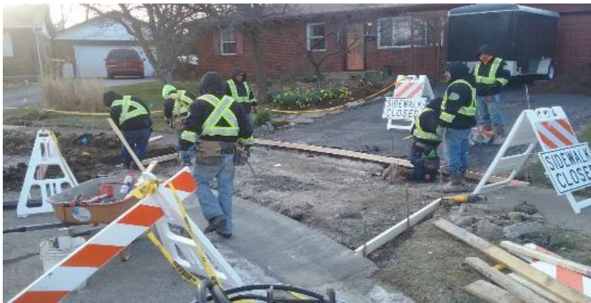
Forming driveway approach in the Cul-de-saq at 421 St. John's Court.
