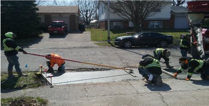
Finishing the driveway approach at 518 St. John's Court.
