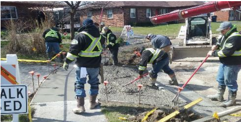
Pouring driveway approach in the Cul-de-saq at 417 St. John's Court.
