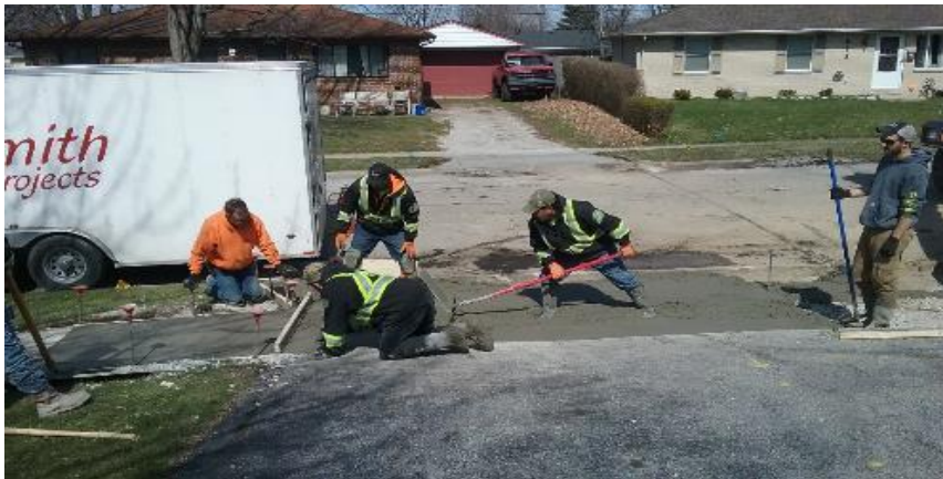
Finishing the driveway approach at 515 St. John's Court.
