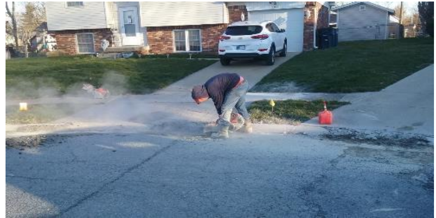
Saw cutting driveway approach in the Cul-de-saq at 502 St. John's Court.
