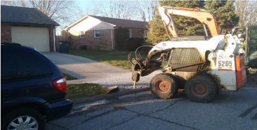
Hammering out curb in the Cul-de-saq at 417 St. John's Court.
