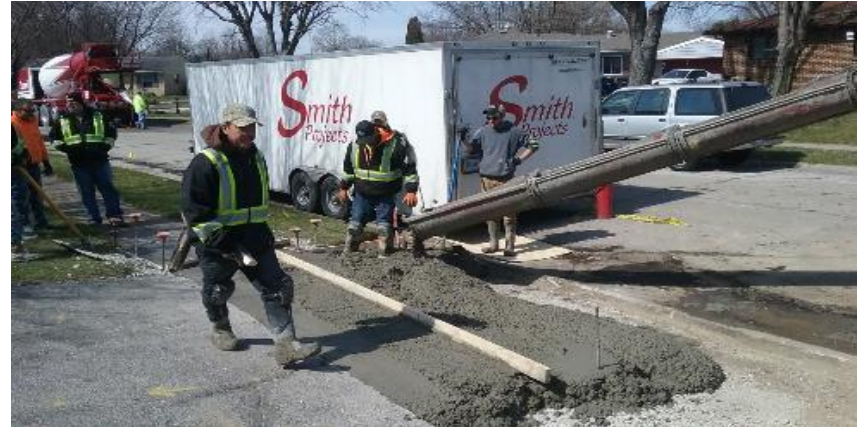
Pouring driveway approach at 515 St. John's Court.
