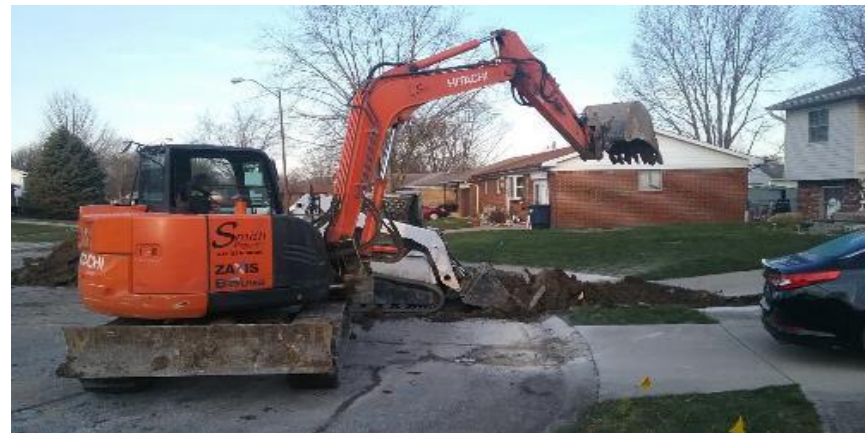
Excavating driveway approach in the Cul-de-saq at 502 St. John's Court.
