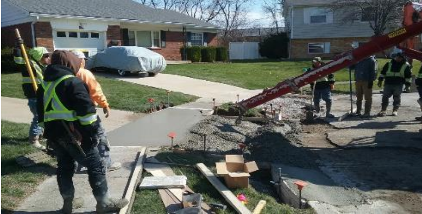
Pouring driveway approach in the Cul-de-saq at 502 St. John's Court.
