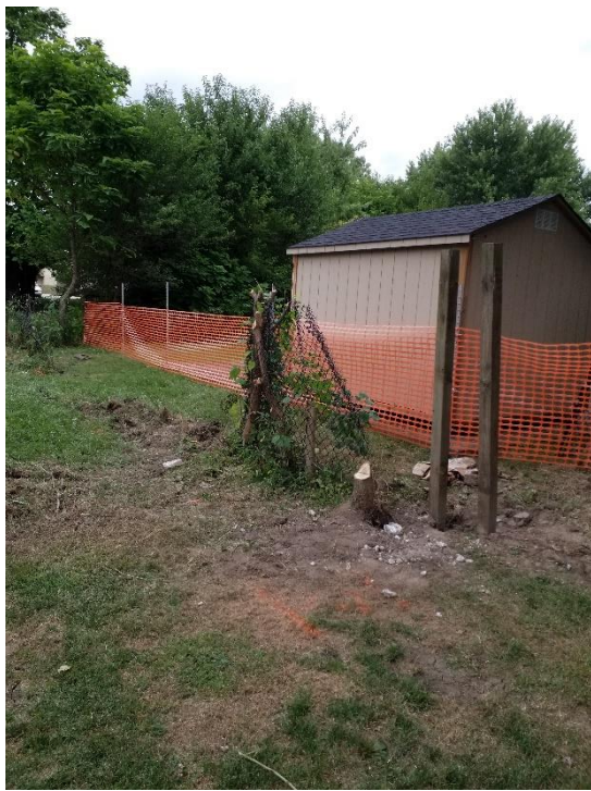
Temporary Fence in Place
