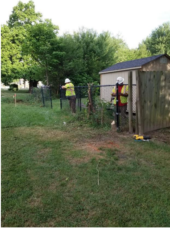
Removing Chain Link Fence
