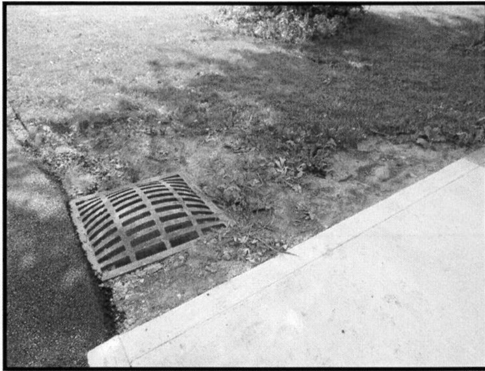
Restore grass around Inlet 22
