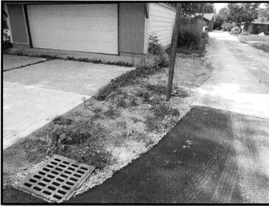
Restore grass area around Inlet 21
