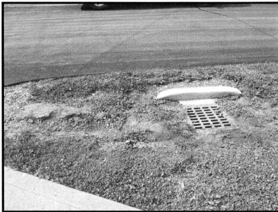
Restore grass around Inlet 24
