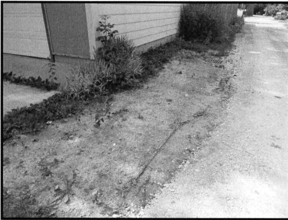
Restore grass area from Inlet 21 to Catch Basin 20
