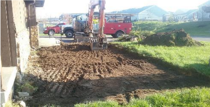
Excavating for ADA ramp on the Henthorn property.
