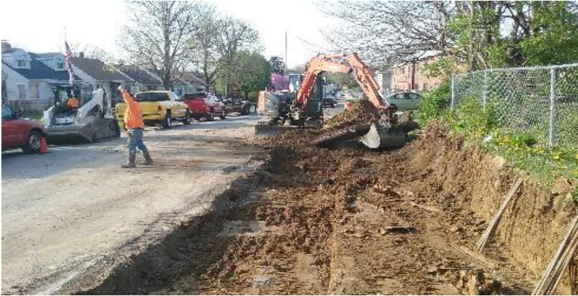
Excavating for sidewalk and curb on the westside of 9th Avenue.
