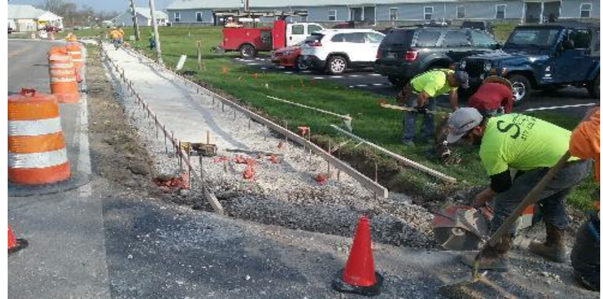
Forming the sidewalk driveway transition at the fire station parking lot.
