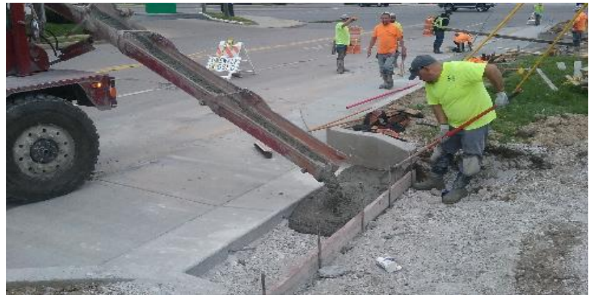
Pouring concrete approach at Henthorn property, northside of Churchman Ave.
