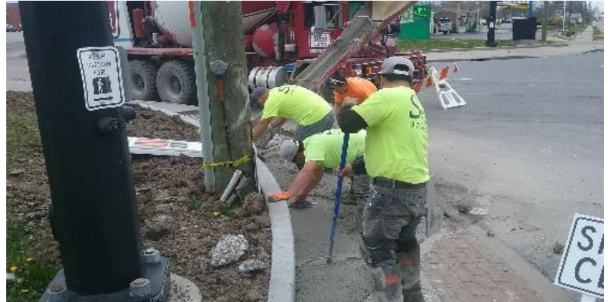
Pouring and finishing concrete sidewalk, corner of Emerson and Churchman.
