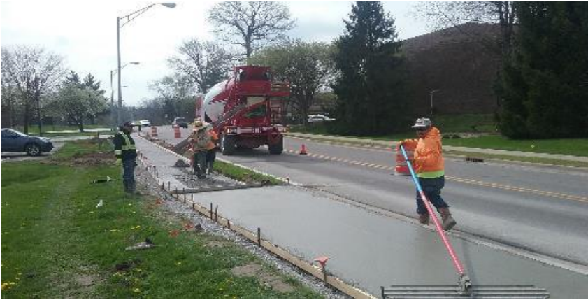
Finishing concrete sidewalk east of Senior facility northside of Churchman Ave.
