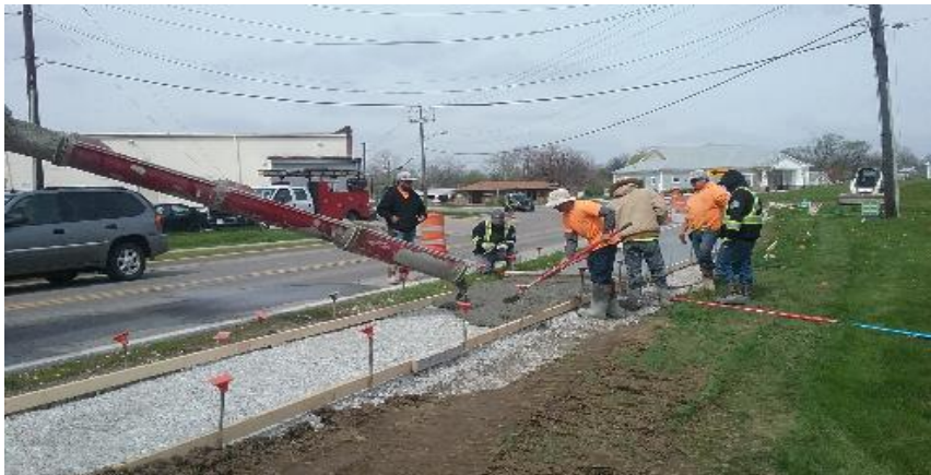
Pouring concrete sidewalk east of Senior facility northside of Churchman Ave.
