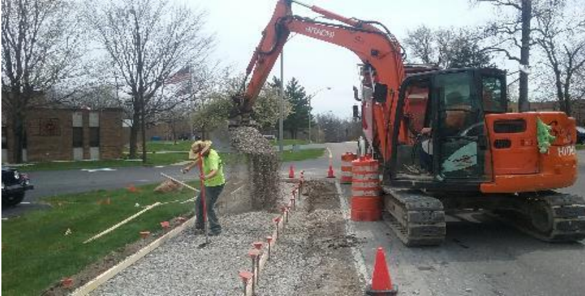
Placing stone for sidewalk subgrade, northside Churchman Ave. at fire station.
