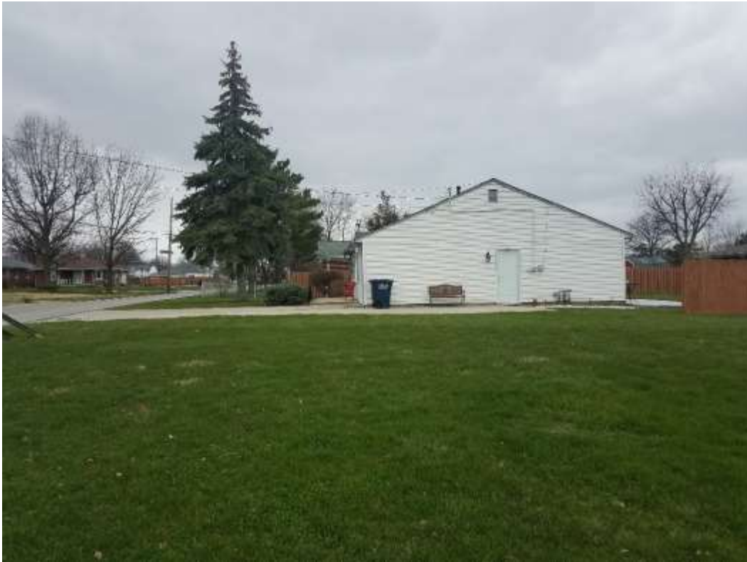
9. Adjacent to west
