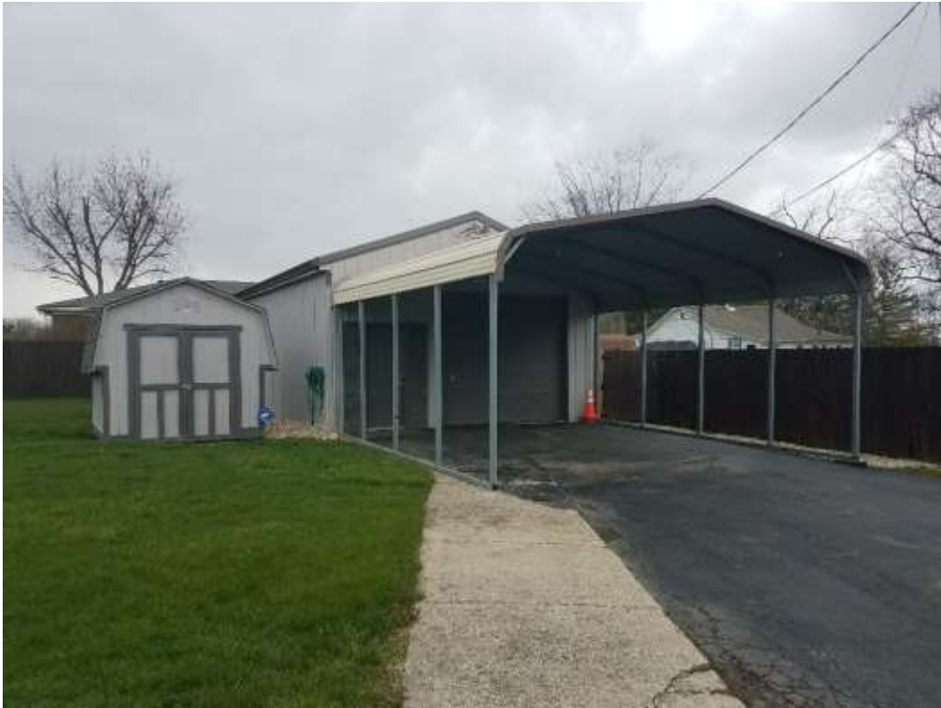
7. Accessory structures on northwest portion of site
